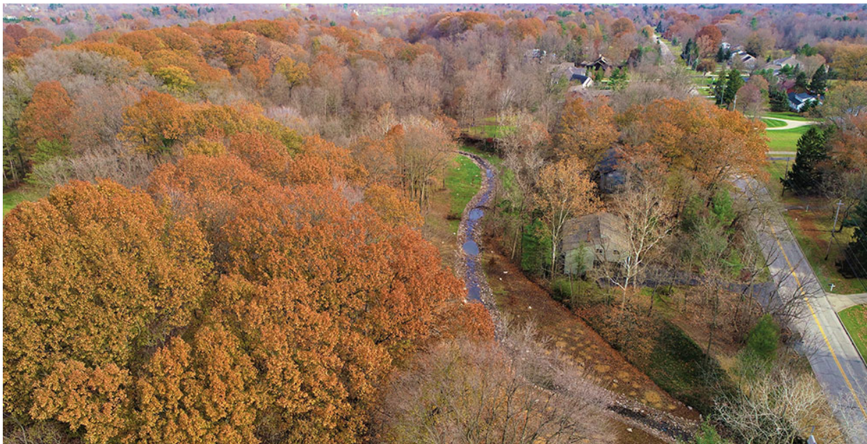
The Pepper Creek development in Pepper Pike restored a creek to help with flood mitigation.
