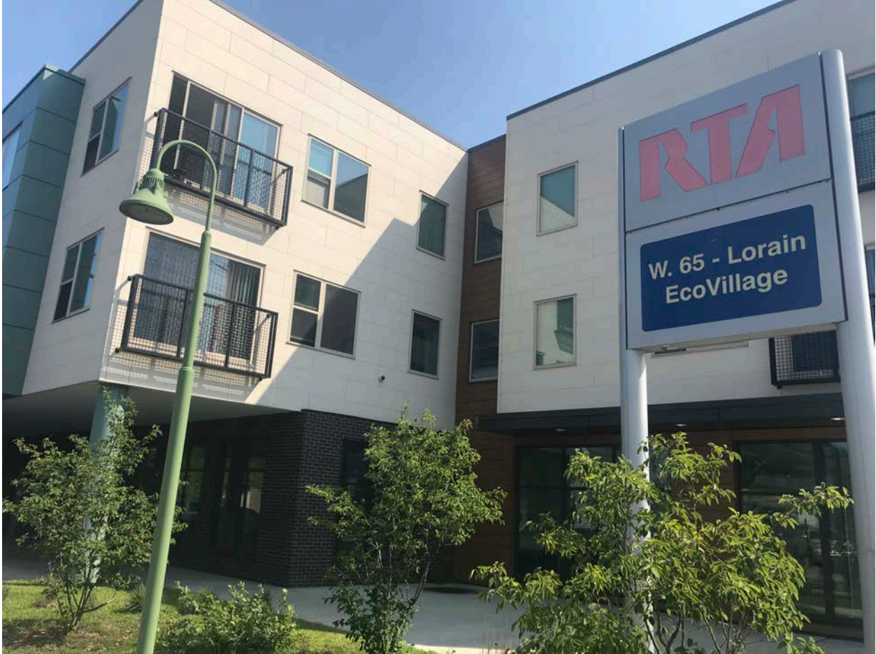
A green-built affordable housing development next to Cleveland's W. 65th Rapid Station
