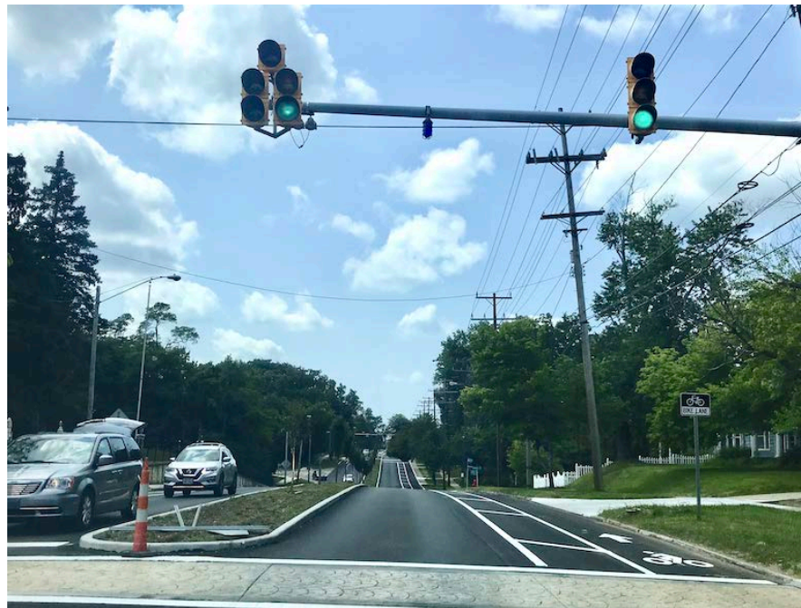
A 'road diet' in Parma Heights led to a planted median and bike lanes
